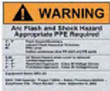
Figure 6 — Equipment Specific Field Label
